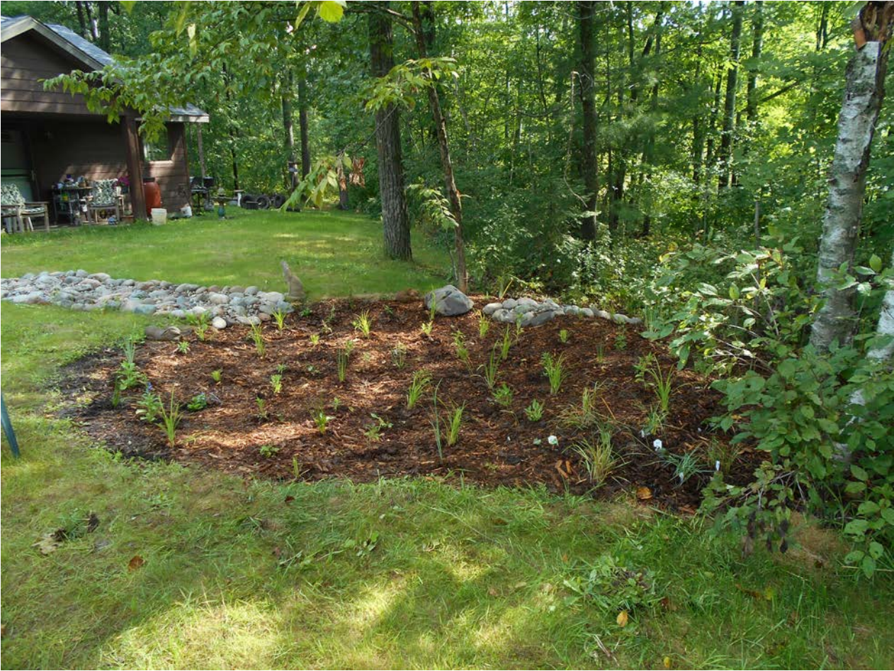
A rain garden was installed near Borden Lake. Stormwater from the home and driveway will be captured.
